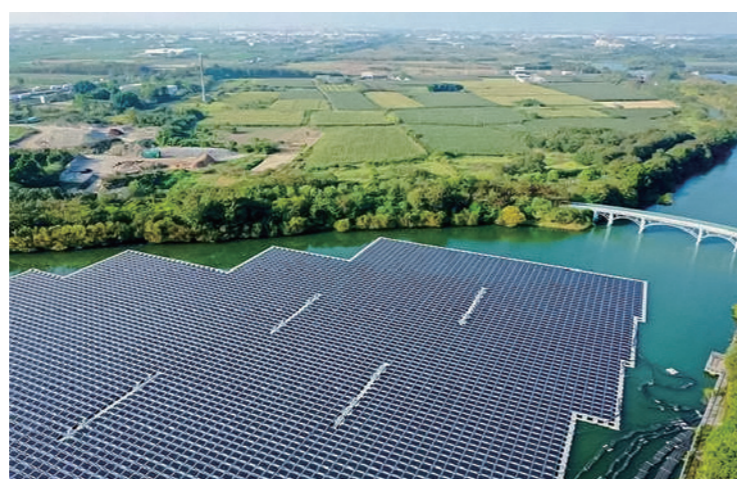
Sugu No. 1 Power Station (4,023kW) Construction of a floating solar power generation system.
