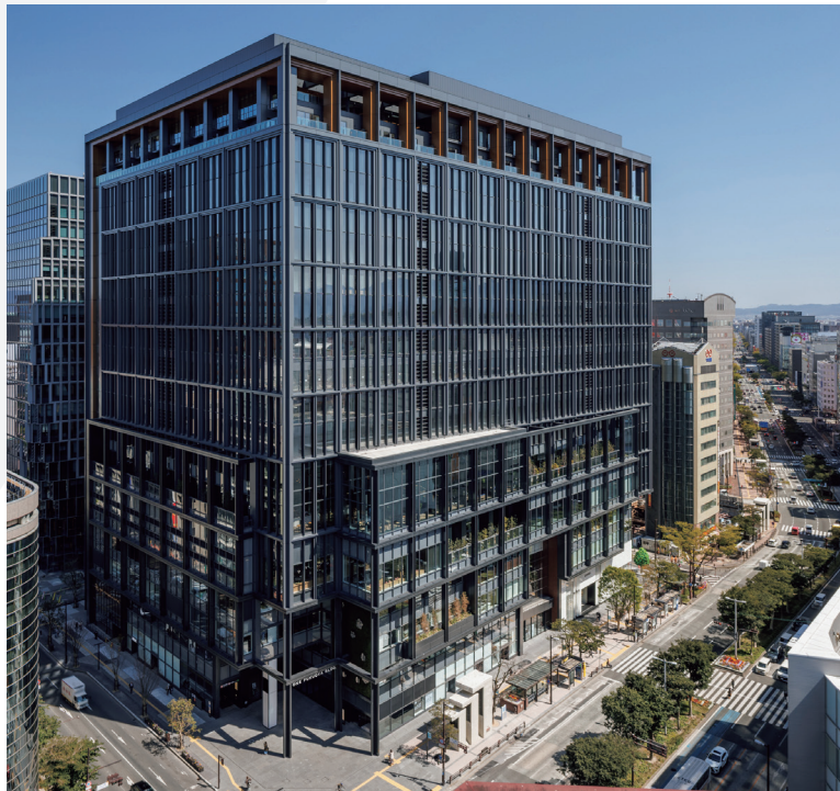
ONE FUKUOKA BLDG. Electrical Work HVAC Work
