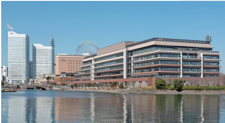
Yokohama Shinko Government Office Building HVAC Work
