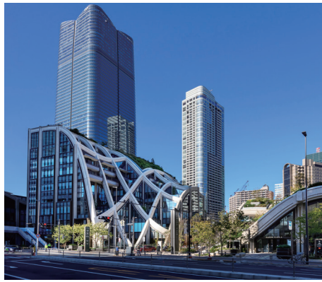
AZABUDAI HILLS Electrical Work
