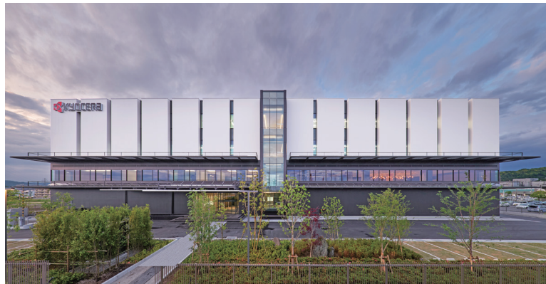
Kirishima R&D Center, Kyocera Corporation Photo by Tomoyuki Kusunose HVAC Work
