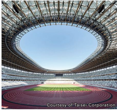
Japan National Stadium Electrical Work
