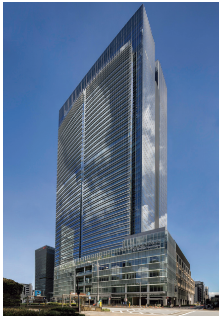
Tokyo Midtown Yaesu Electrical Work
