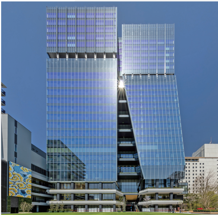
Fukuoka Daimyo Garden City HVAC Work
