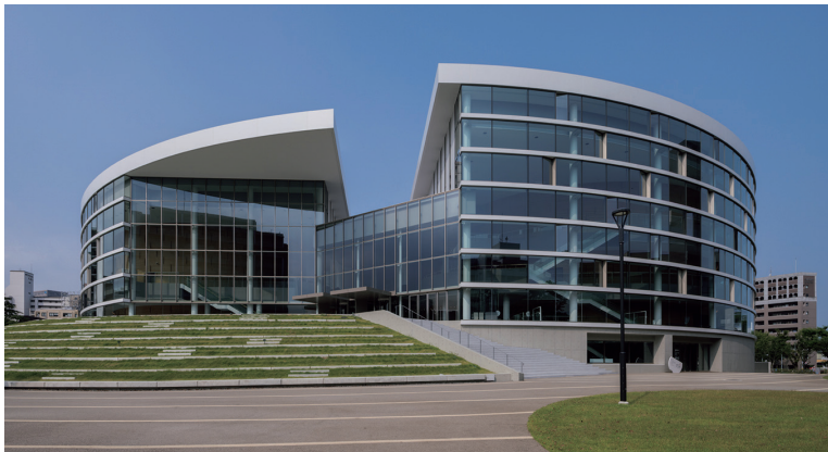
Fukuoka Civic Hall Photo by Yousuke Harigane Electrical Work
