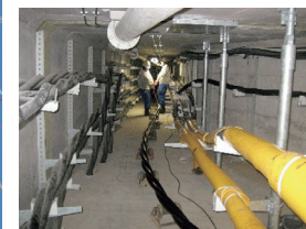
Cable laying work
