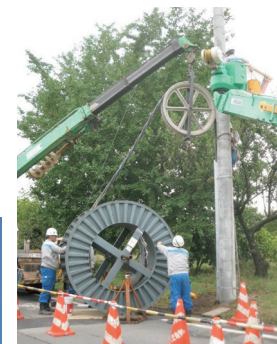
Cable feeding work
