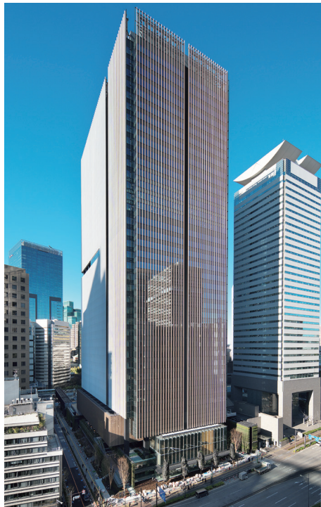
Toranomom Alcea Tower HVAC Work
