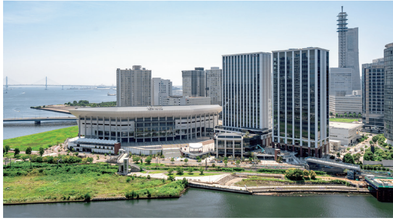
K-Arena Yokohama Electrical Work
