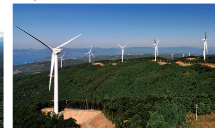
Kushima Wind Power Generation Plant
