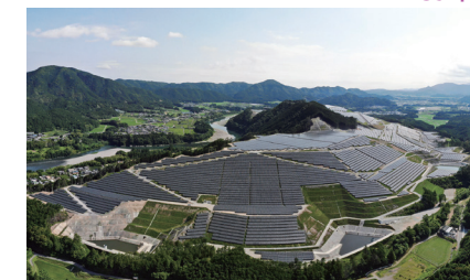
Miya River Watarai Solar Park
